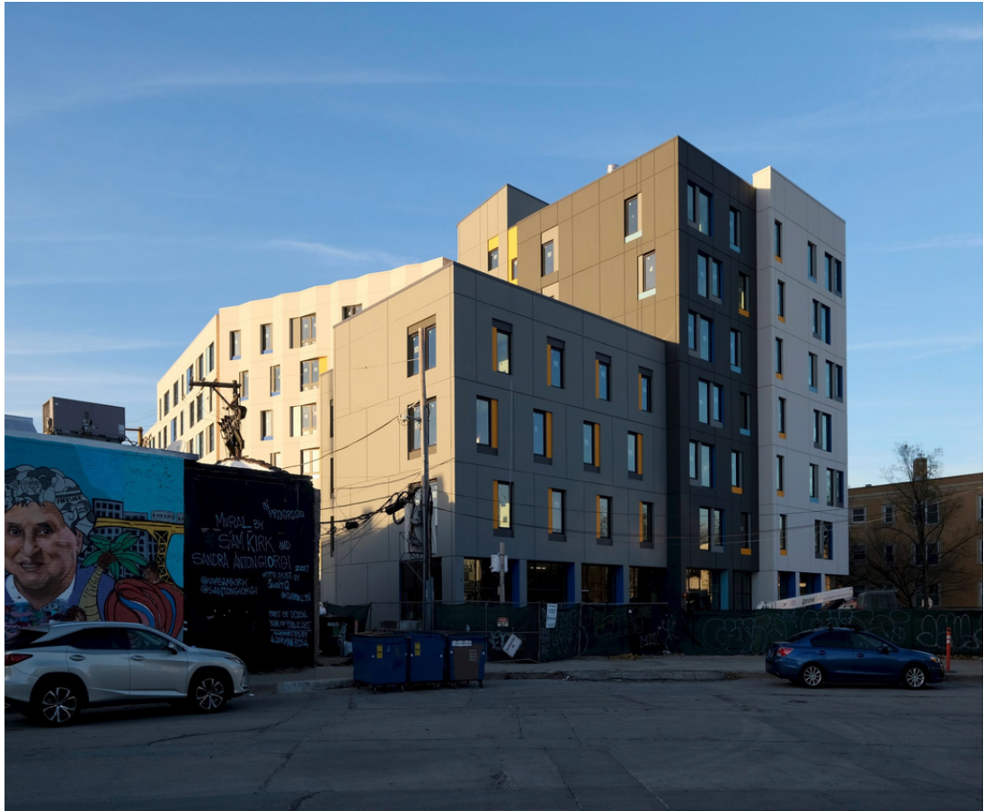
Emmet Street Apartments, a Chicago LIHTC Development that opened in 2022 with 100 affordable units.
