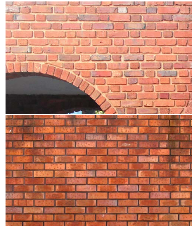
Flemish Bond (upper left), Stretcher Bond (lower left), Belk Library Detailing (upper right), and Inman Admissions Detailing (lower right)
