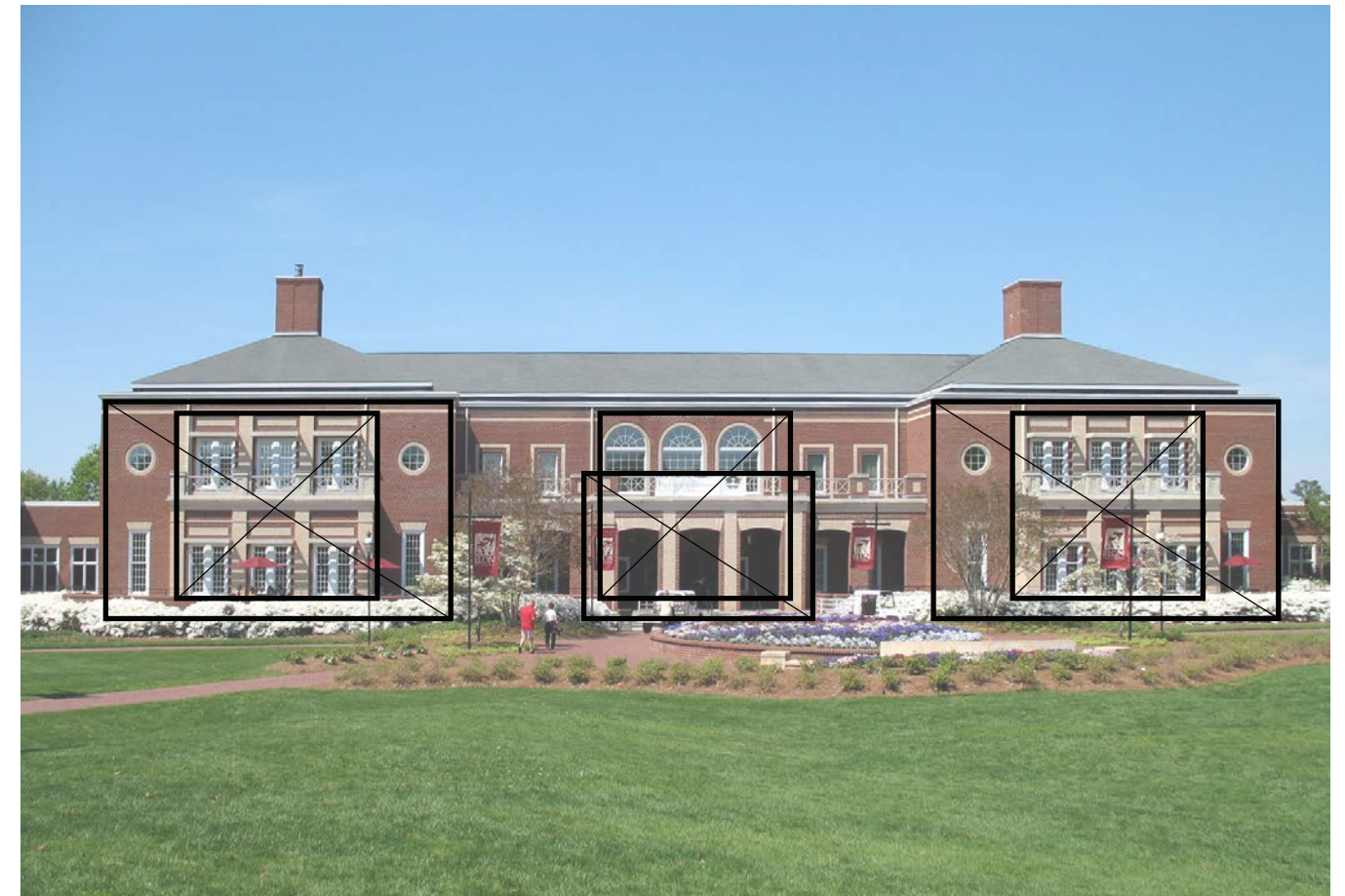
Common Proportions at Moseley Center
