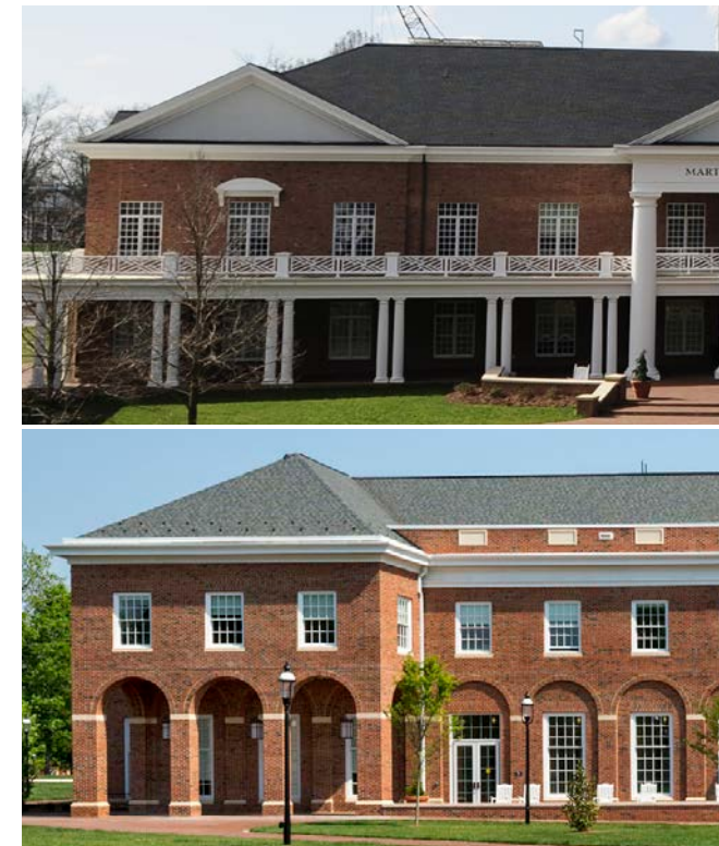
Mixed Gable and Hip Roof Form, Lindner Hall (upper left), Hip Roof Form, Inmand Admissions (lower left), and Schar Hall Cupola (right)
