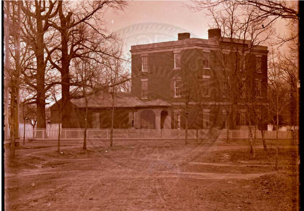
"Unidentified building" (most likely the South faculty residence). Source: UM Special Collections, Edward C. Boynton Collection (circa 1860)
